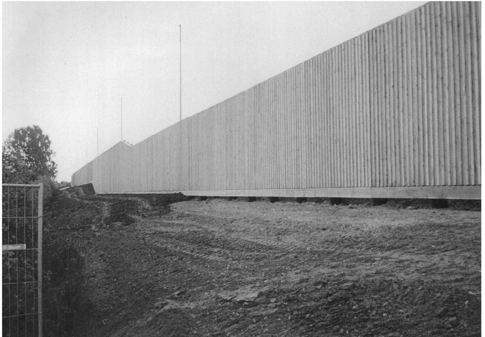
The structures can be pre-fabricated or site built depending upon factors such as rapid build or restricted site access. They are also lightweight structures compared with concrete or block which require foundations.
