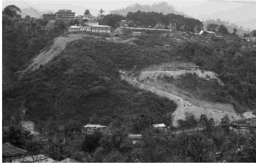
Figure 9. A stabilized hill slope being disturbed by construction of houses, below Banquet Hall, Itanagar, March 2002.
