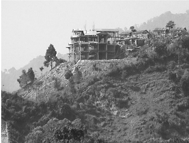
Figure 10b. Closer view of the Figure 10a, showing the building under high risk, February 2005.
