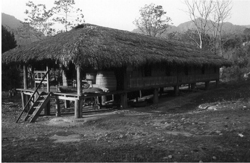
Figure 13. A traditional house in Arunachal Pradesh made of wood and bamboo with palm leaf roof, March 2002.
